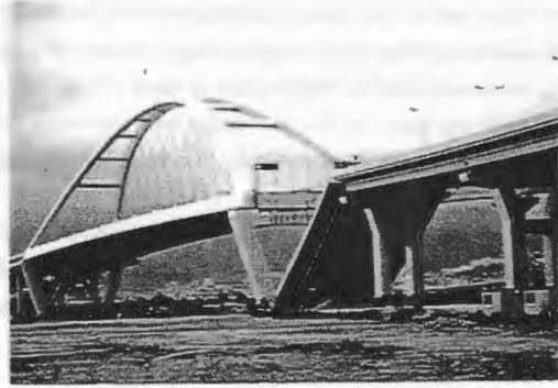
Photo 5 Unseating, side span of the Nishinomiya bridge
